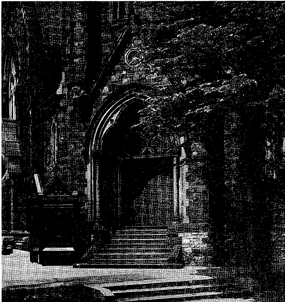
A PHOTOGRAPHIC STUDY OF THE TOWER ENTRANCE OF JARVIS STREET CHURCH.
