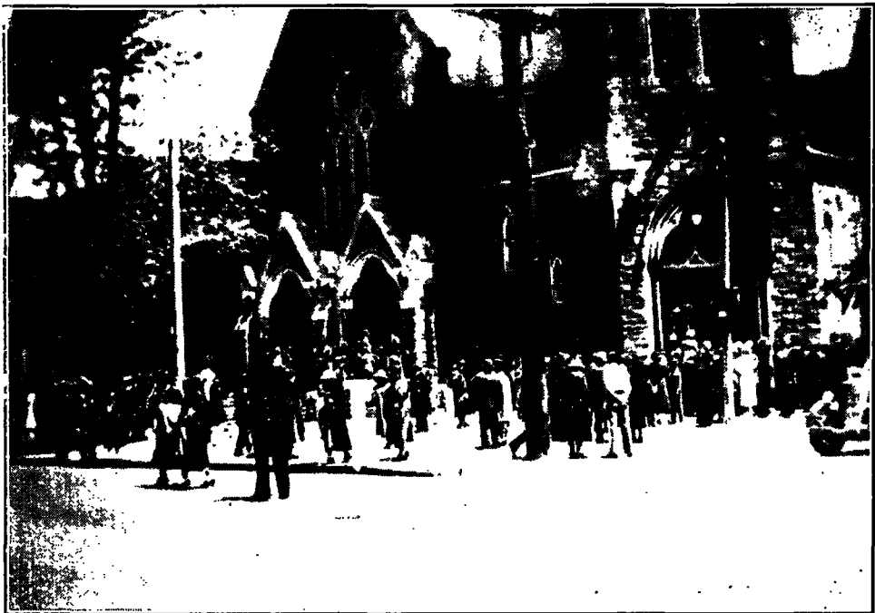
VIEW OF THE MAIN AND SOUTHWEST ENTRANCES
