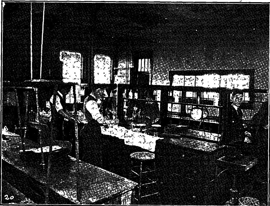
Advanced Chemical Laboratory.
